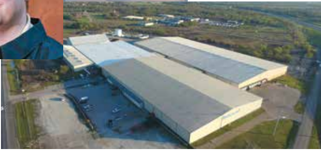
Polyguard's facility in Corsicana, Texas
